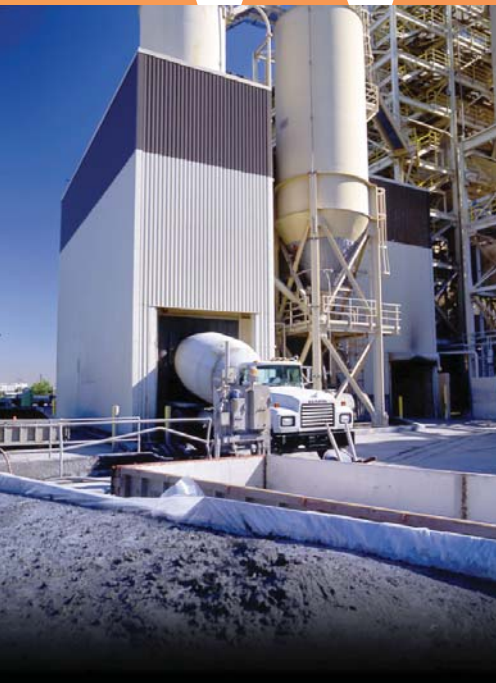
Commerce Waste-to-Energy Facility
